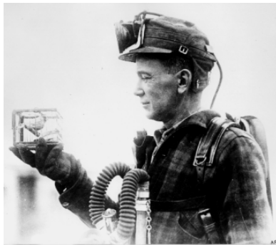
Small cage with canary bird used in testing for carbon monoxide gas in Hollinger Mine, Timmons, Ontario, Canada. ( http://www.msha.gov )
